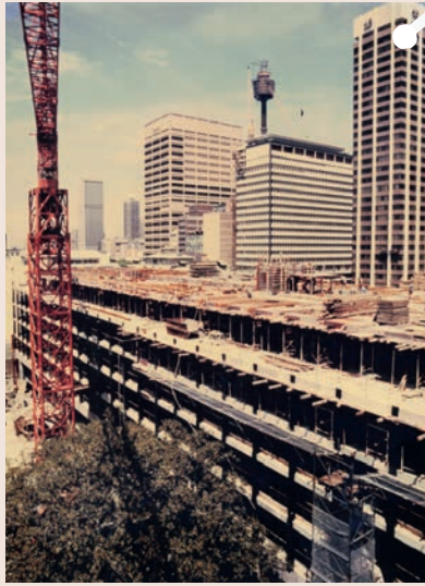
CONSTRUCTION OF TOWER BLOCK PARLIAMENTARY COLLECTION
