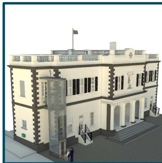
Plans for an addition of an external elevator to the Parliament of Gibraltar, source:
